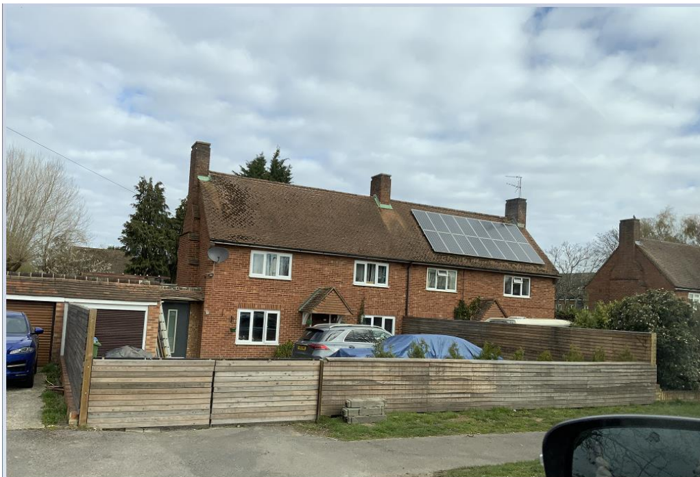
Figure 1: The site following compliance with the Enforcement Notice
